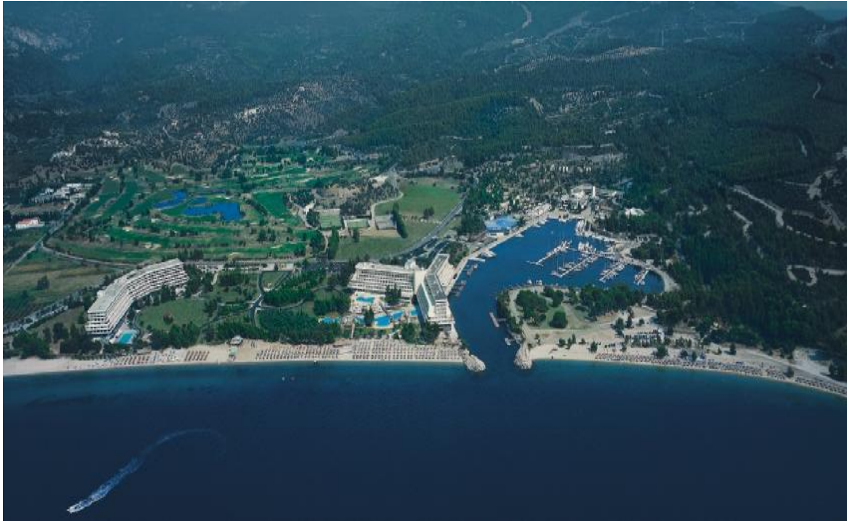
Partial Aerial Overview
