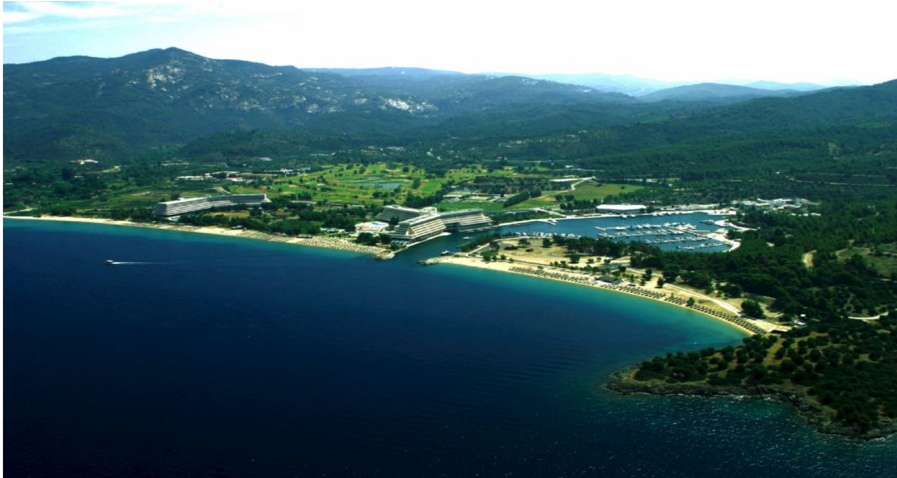
Partial Aerial Overview
